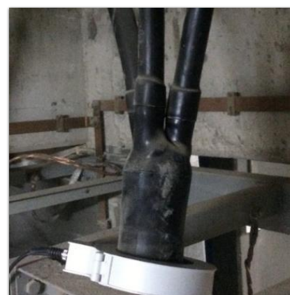
Trifurcating termination replaced
